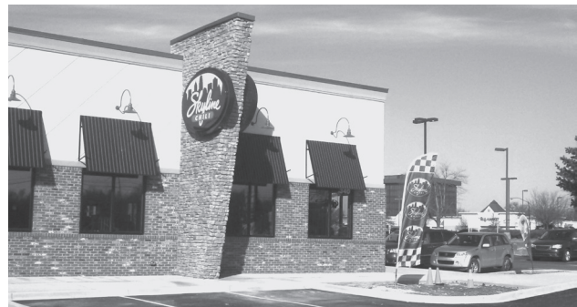
New Site located off Whittington Pkwy – facing Hurstbourne
